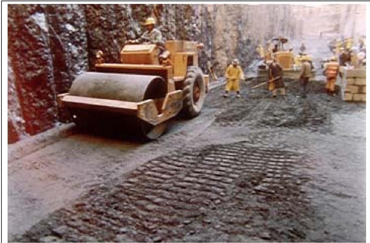
**Foundation RCC Backfill at Itaipu Diversion Chanel-1978**
