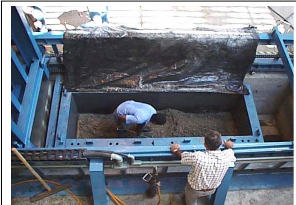
**Levelling the RCC Layer**
