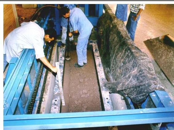
**Measuring the RCC layer height and compaction close near the form**
