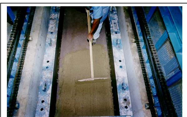
**Bedding mortar spreading at RCC Joint**
