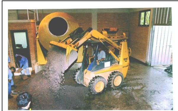
**Mix homogenization with a front loader machine**
