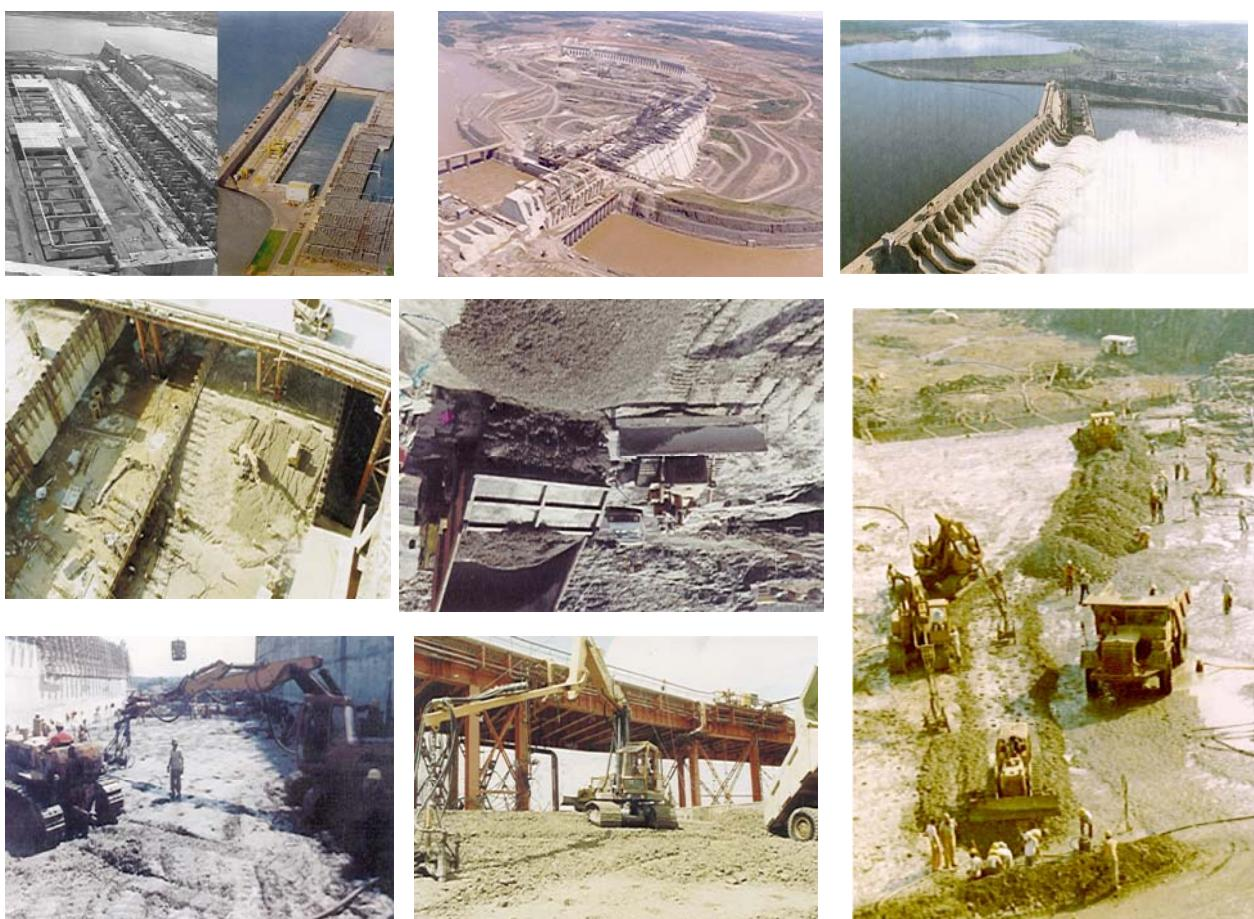
**Brazilian Dam where have been used Conventional Mass Concrete with cementitious content less than 100kg/m<sup>3</sup>**
