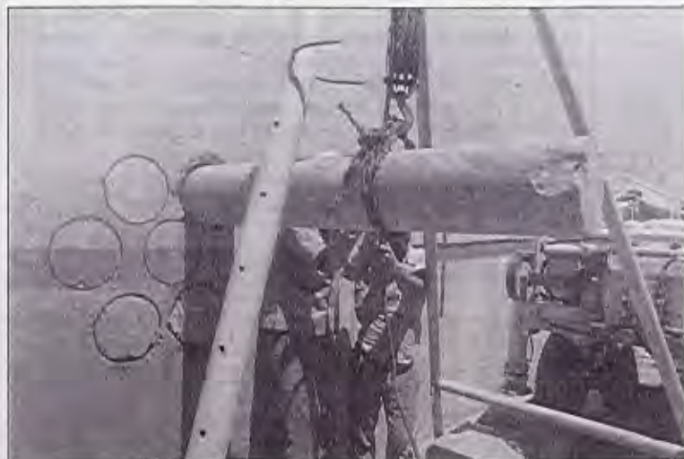
Drilling cores at Itaipu.
