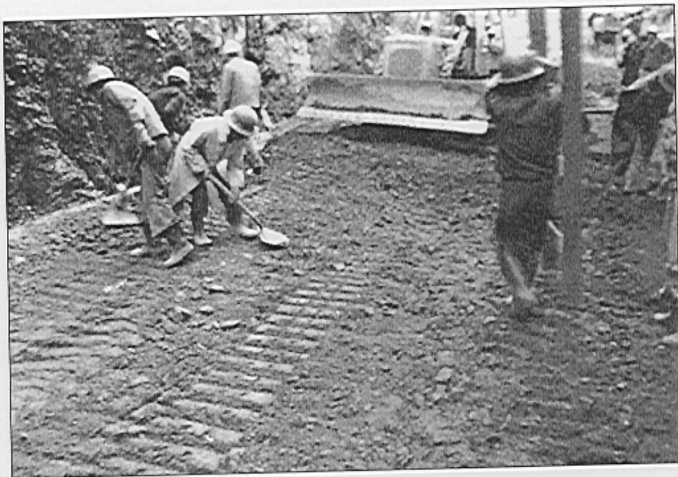
FIGURE 2- RCC USED FOR BACKFILLING A ACCESS RAMP AT ITAIPU DIVERSION STRUCTURE (1978)
