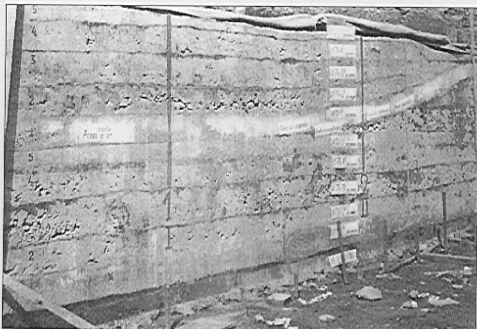
FIGURE 3-EXPOSED SURFACE, CASTED WITH FORMWORKS, AT ITAIPU TESTFILL (1979)
