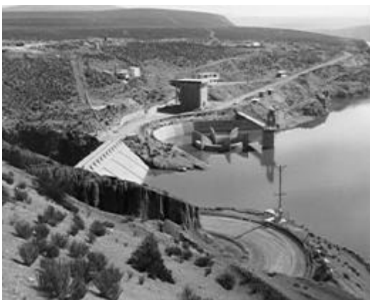
Figure 3 - View of the Aguada Blanca dam
