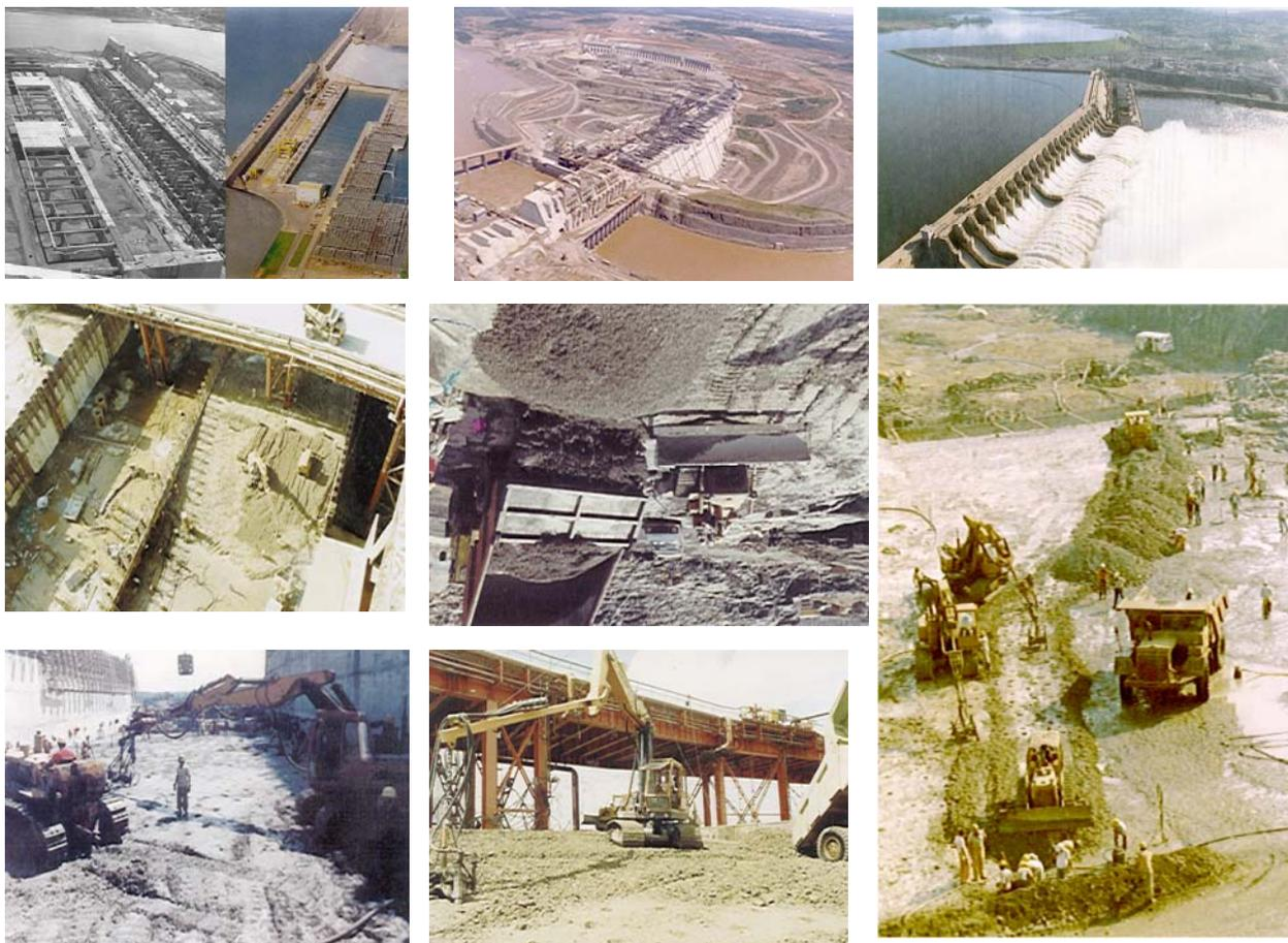
**Brazilian Dams where have being used Conventional Mass Concrete with cementitious content less than 100kg/m<sup>3</sup>.**
