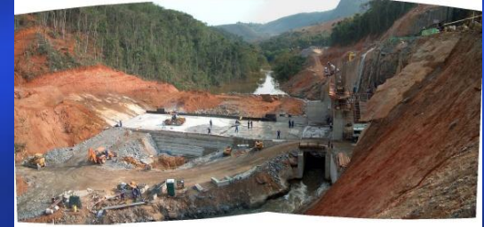
Picada – Double curvature formwork (II)
