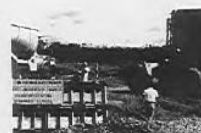
Rollercrete was applied to a permanent structure for the first time in Brazil at the Tucuruí Dam navigational lock.
