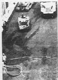
General view of rollercrete placement at the Itaipu project.
