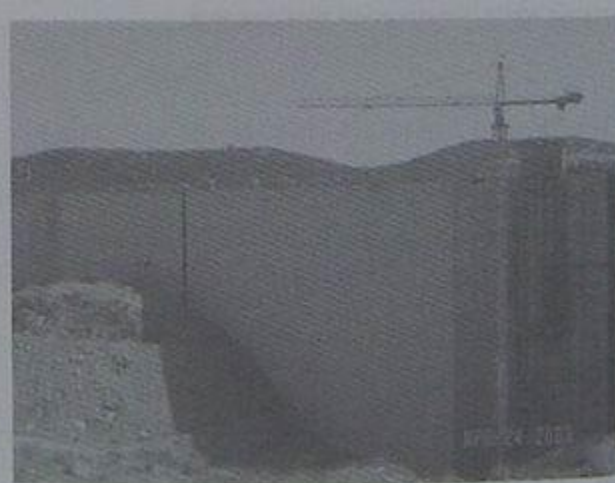
Figure 9. Olivenhain, USA: the PVC geocomposite under installation at left abutment.
