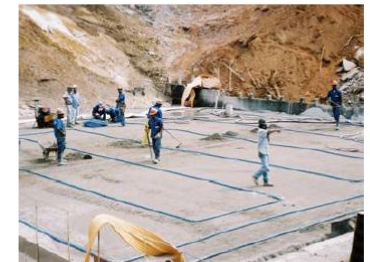
Picada – Post-cooling system
