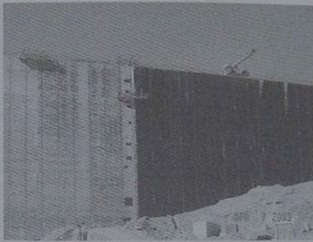
Figure 8. Olivenhain, USA: the drainage geonet is placed on the RCC and under the PVC geocomposite to enhance drainage collection and discharge.
