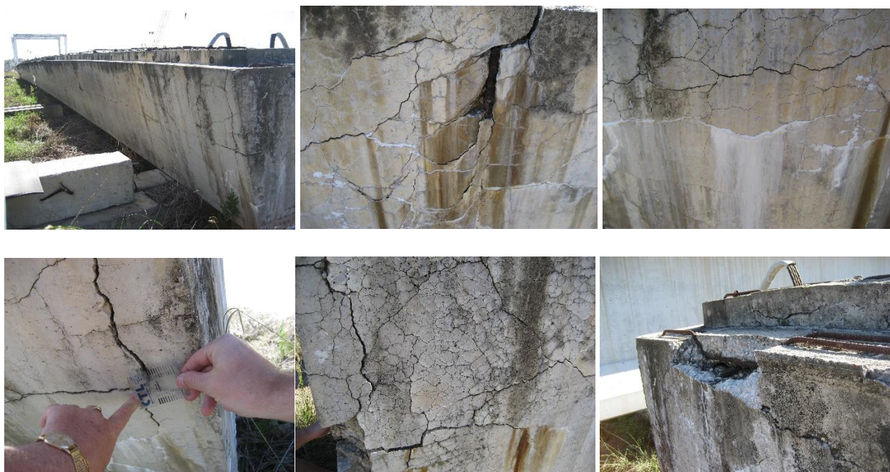
Figs. 6 – Concrete precast beam steam cured in a temperature greater than 70^\circ\text{C} , and the scenario of cracks due to DEF.
