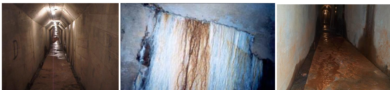
Figs. 5 – A gallery in a Dam; the leakage in a construction joint ad the sediment with a brown-red color inducing the sulfate [3]
