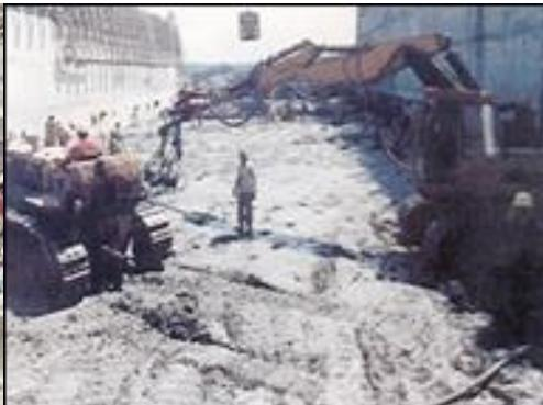
Conventional Vibrated Mass concrete poured by buckets handled by cable way, spread by frontal blade tractor and vibrated by a gang of four vibrators hanged by a backhoe excavator - 1977-Itaipu
