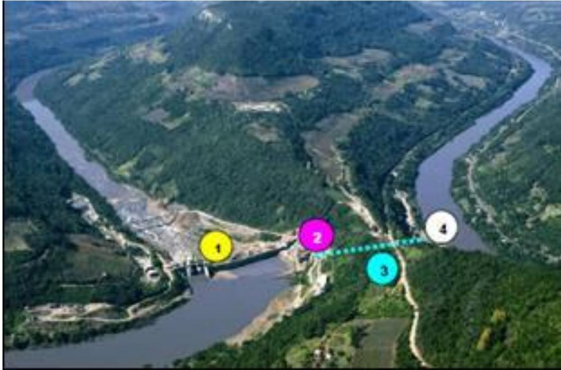
1-RCC Dam and Spillway
