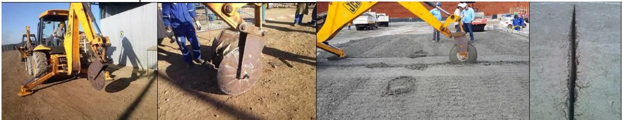
**A new, and simple approach to cast the contraction joint, adopted recently in a RCC Dam in Brazil**
