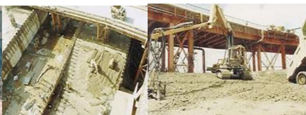
Sloped pouring used at Tucurui construction for CVC mass concrete- 1981
