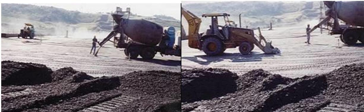
**Bedding mortar being applied on the surface of RCC construction Joint**
