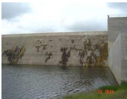
**Leakage due to mistakes in the face concrete**
