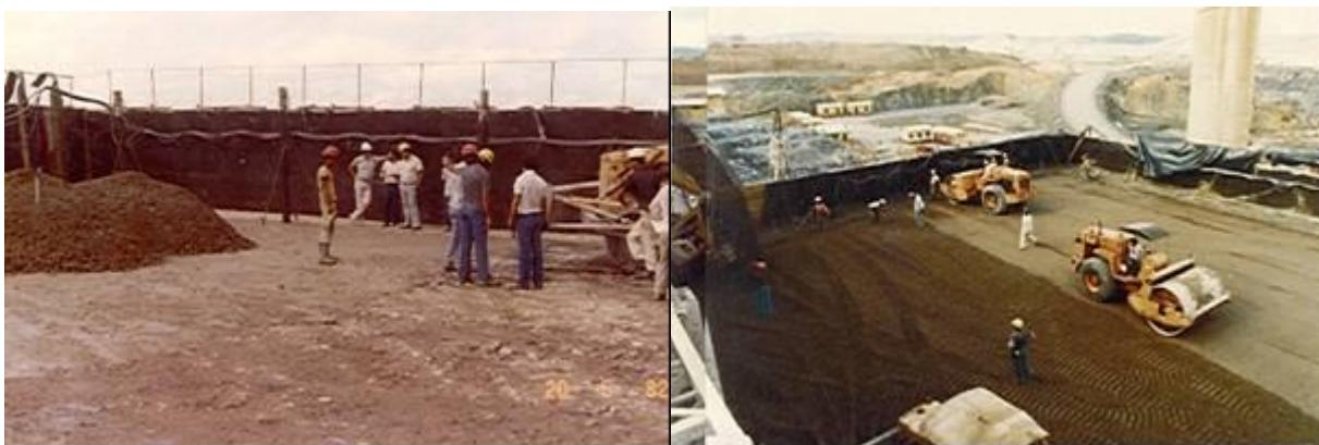
RCC being poured in a block of the navigation lock at Tucurui Dam – 1982
