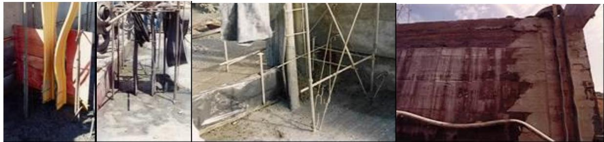
Double line of PVC water-stops, drain and the aspect of the face at contraction joint with the water-stop
