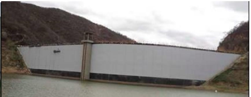
**Repair at Saco de Nova Olinda, by applying a PVC membrane by 2011/2012, about 25 years after the construction**
