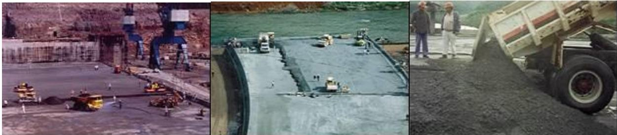
RCC placement by extensive horizontal layers, considered the traditional method
