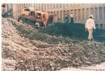
Sloped pouring used at Itaipu construction for CVC mass concrete-1977
