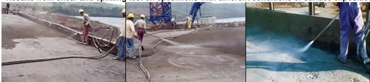
RCC surface cleaning for the subsequent placement with humidity air
