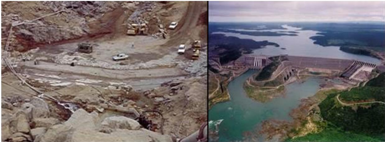
CHESF- RCC Protection of the Rock-fill for overtopping at Xingo CFRDam
