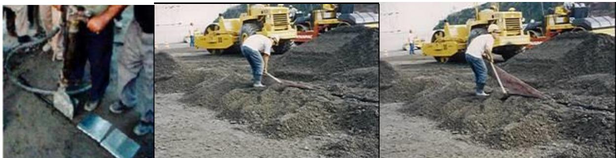
**Casting of the contraction joint, by inserting metal blade with help of hammer break**
