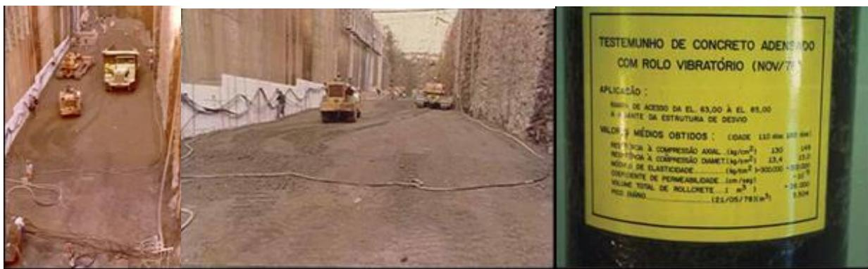
Back filling the access ramp and drilled core from the RCC poured in the access ramp
