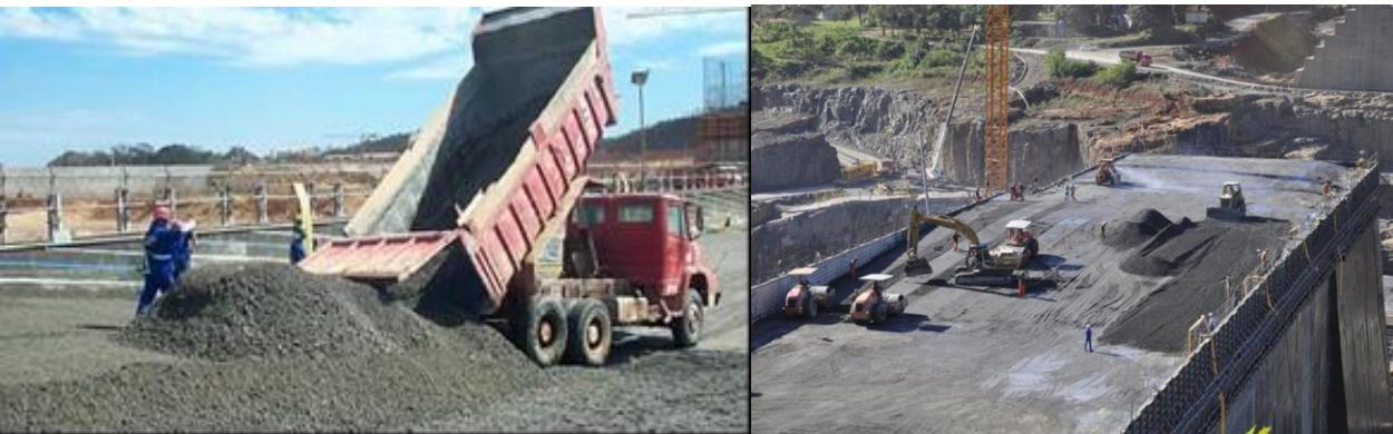
RCC placement using sloped layer method
