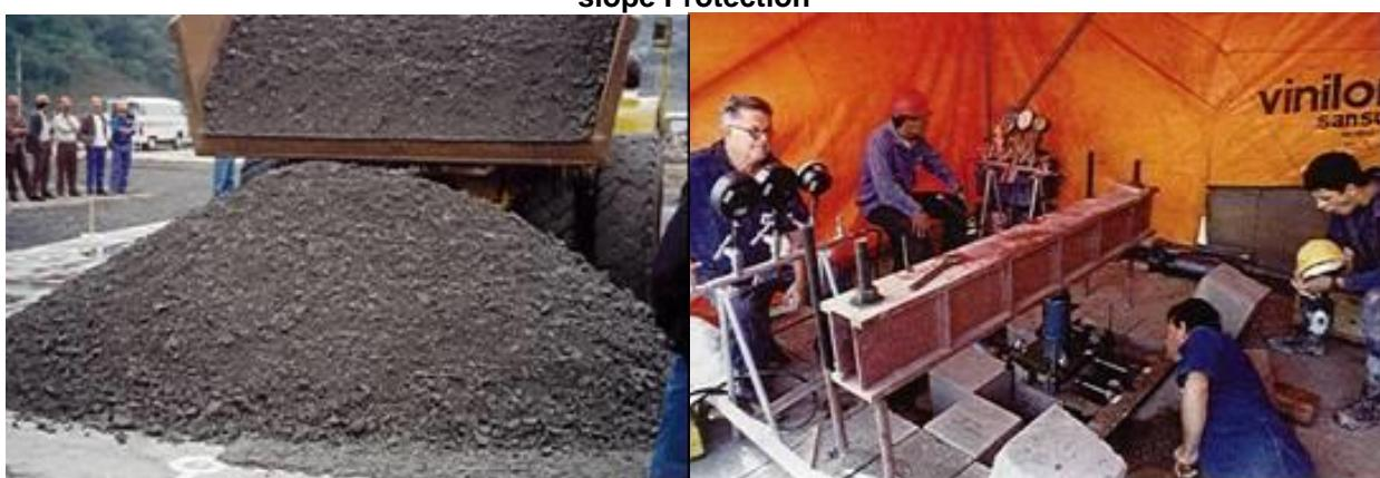
COPEL- A preliminary test fill at Segredo Dam, before Jordao RCC Dam and in situ shear test for Salto Caxias RCC Dam
