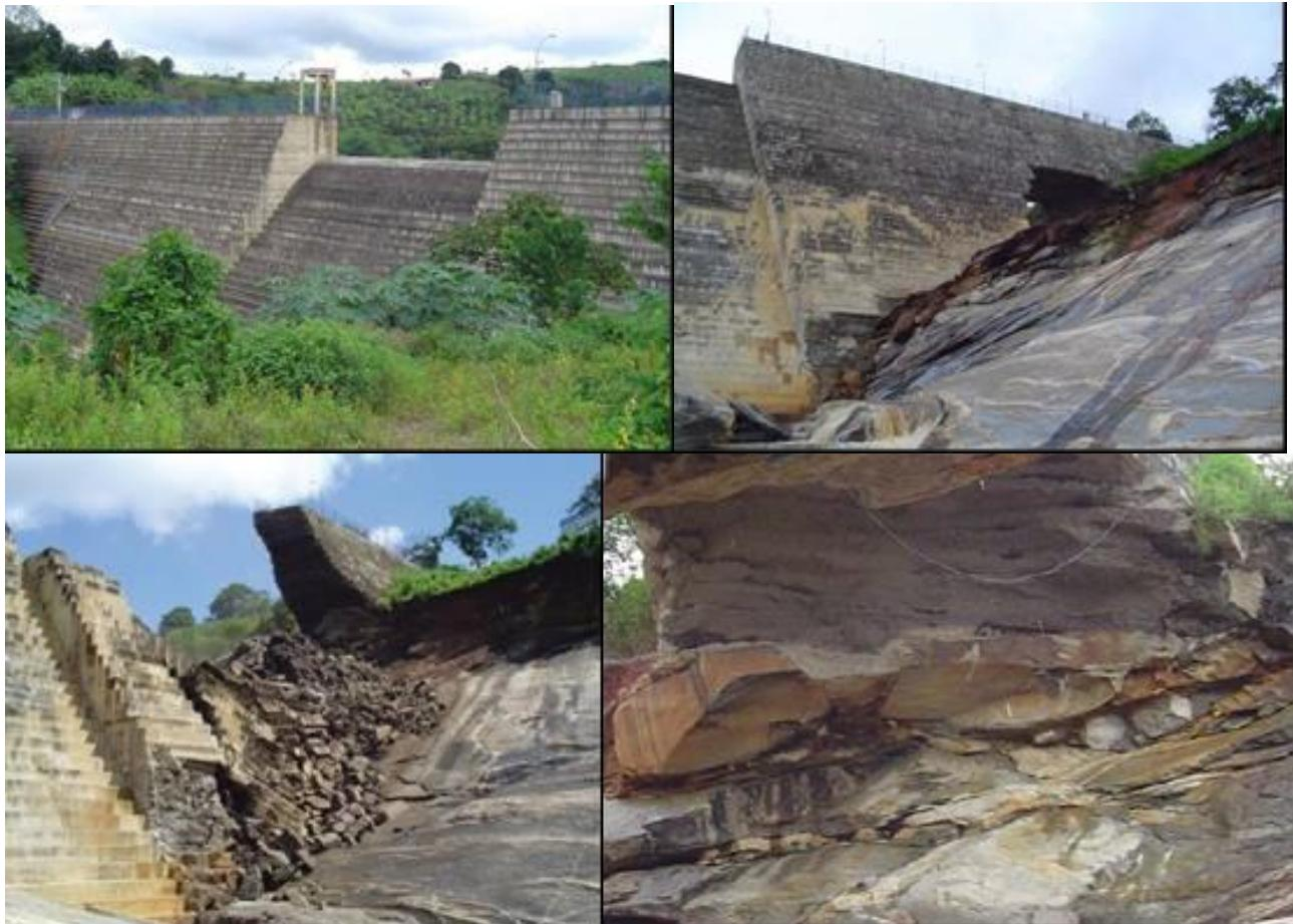
Sequence of the rupture, and the weathered rock and block under the dam contact
