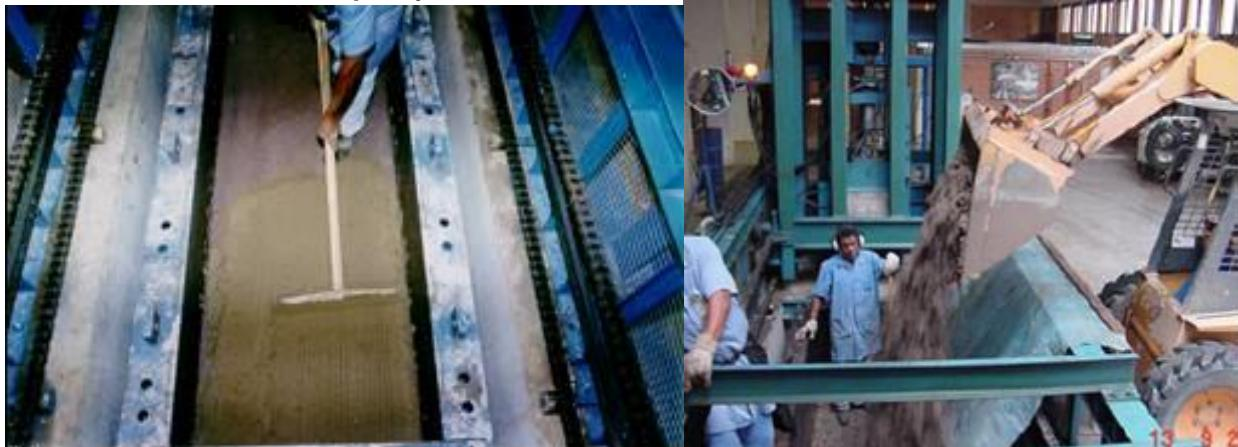
Bedding mortar spreading at RCC Joint
