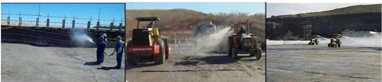
**RCC protection during placement and curing, with different equipment, tool and manner, during Brazilian RCC construction**
