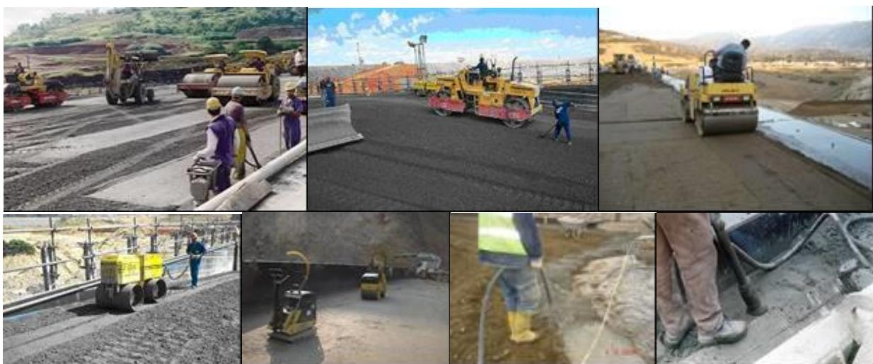
**Compaction rollers of different types, models and sizes, vibratory plate for RCC and immersion vibrator for CVC and/or GeRCC, normally used in Brazil**
