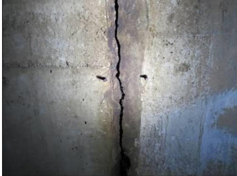
**Aspect of the opening of a Contraction Joint within the dam. The Contraction Joint on an inflection of the foundation of rock mass of high modulus of elasticity**
