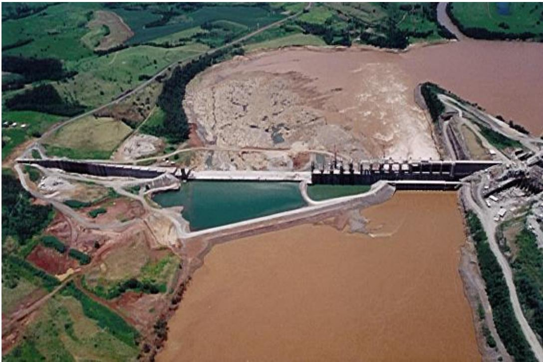
**Salto Caxias during construction- as prepared for a large flow- around 15.000m<sup>3</sup>/s- (7.500m<sup>3</sup>/sec through the sluiceway and 7.500m<sup>3</sup>/sec over the dam under construction)**
