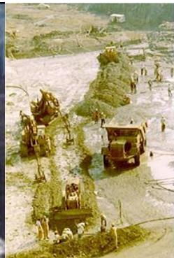
Conventional Vibrated Mass concrete poured, in a large backfilling area, directly by a dump rear of road truck spread by frontal blade tractor and vibrated by a gang of four vibrators hanged by a backhoe excavator - 1978-Itaipu
