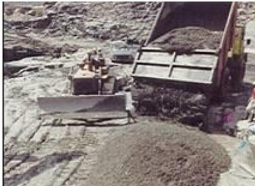
Conventional Vibrated Mass concrete poured directly by a dump rear of road truck, spread by frontal blade tractor and vibrated with immersion vibrators- 1977-Itaipu
